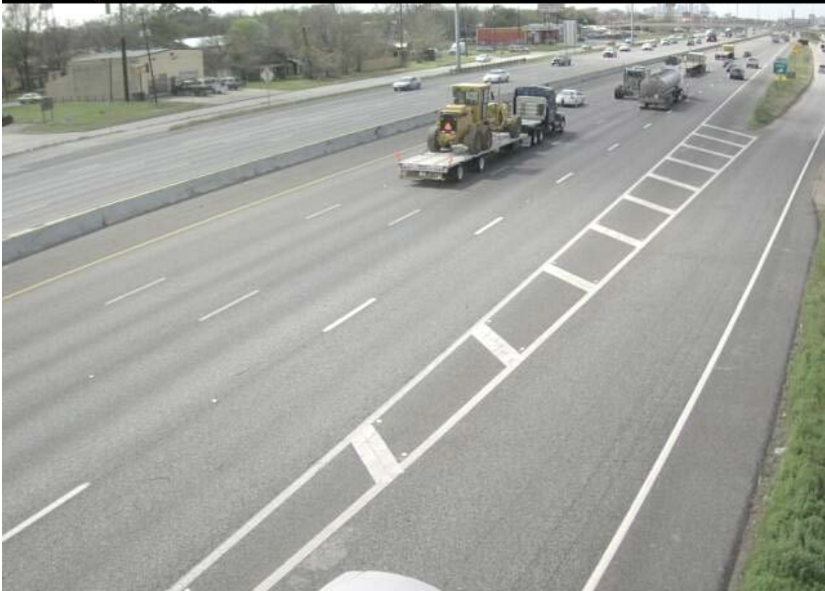
Figure 12. Lowboy Overheight Load at the Mercury Site (continued on I-10 Inside of I-610).
