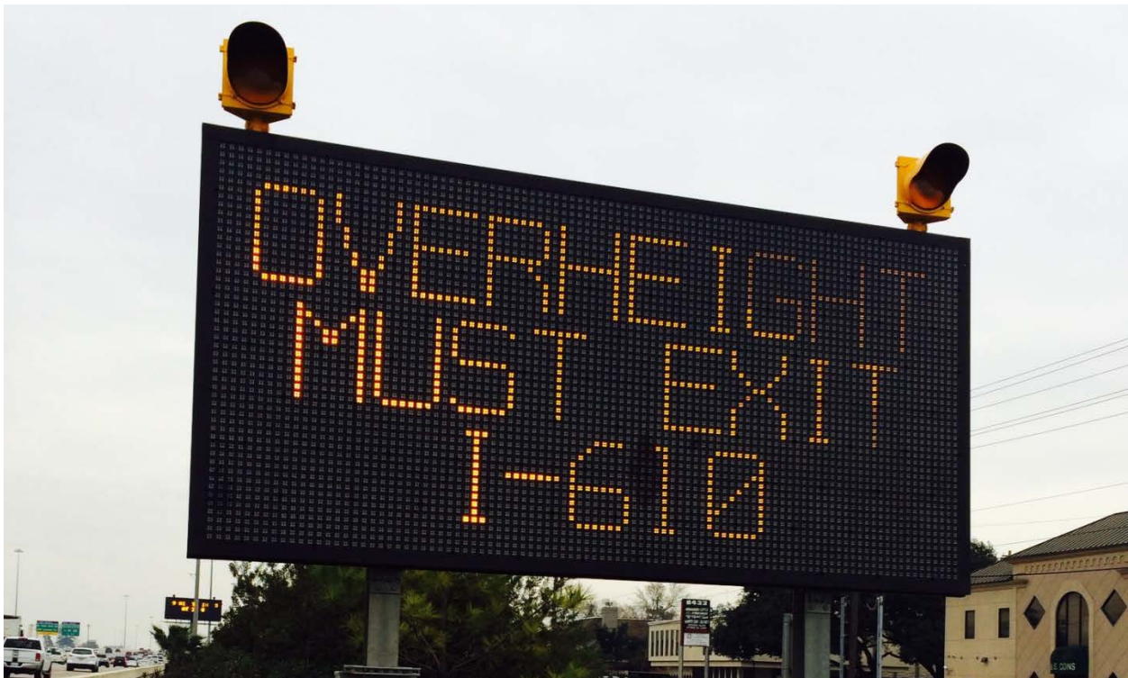
Figure 3. DMS with Top Mounted Beacons Showing the Warning Message.
